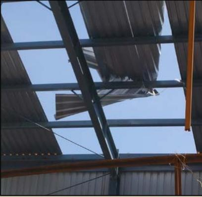
The main damages were found to be trees uprooting, roof damages to non RCC buildings having Kuthca/ACC & metal sheet roofs, road damages due to fall of trees, damages to standing crop.
