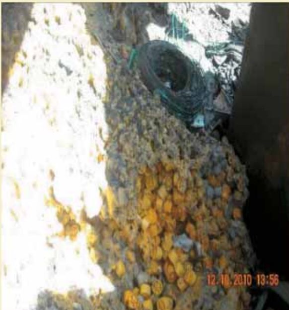
Damaged plastic wheel in the mezzanine floor
